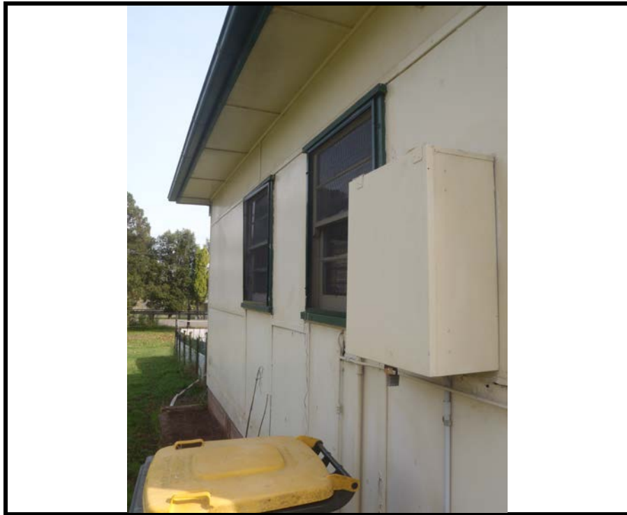
Photo 3: Example of ACM sheeting eaves and exterior walls to 1 Dawes Avenue
