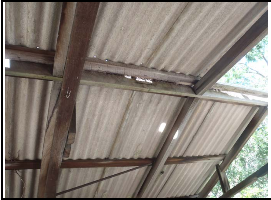
Photo 23: ACM corrugated sheeting used on garage at 4 Dawes Avenue
