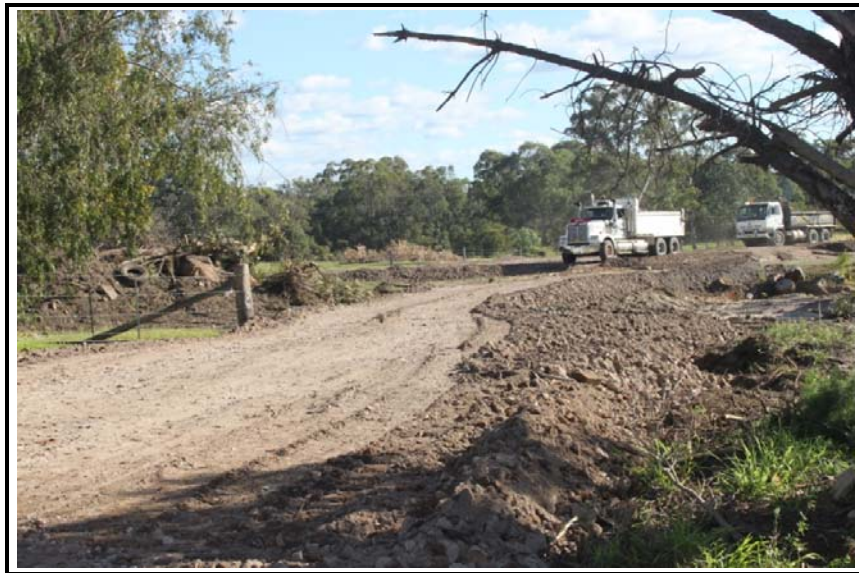
Photo 2: 6/5/14: Imported fill removal in progress at Loxford Fabrications.
