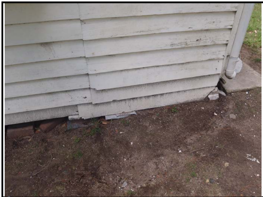
Photo 18: ACM sheeting used in place of weatherboard sheeting at southeast side corner of 2 Dawes Avenue
