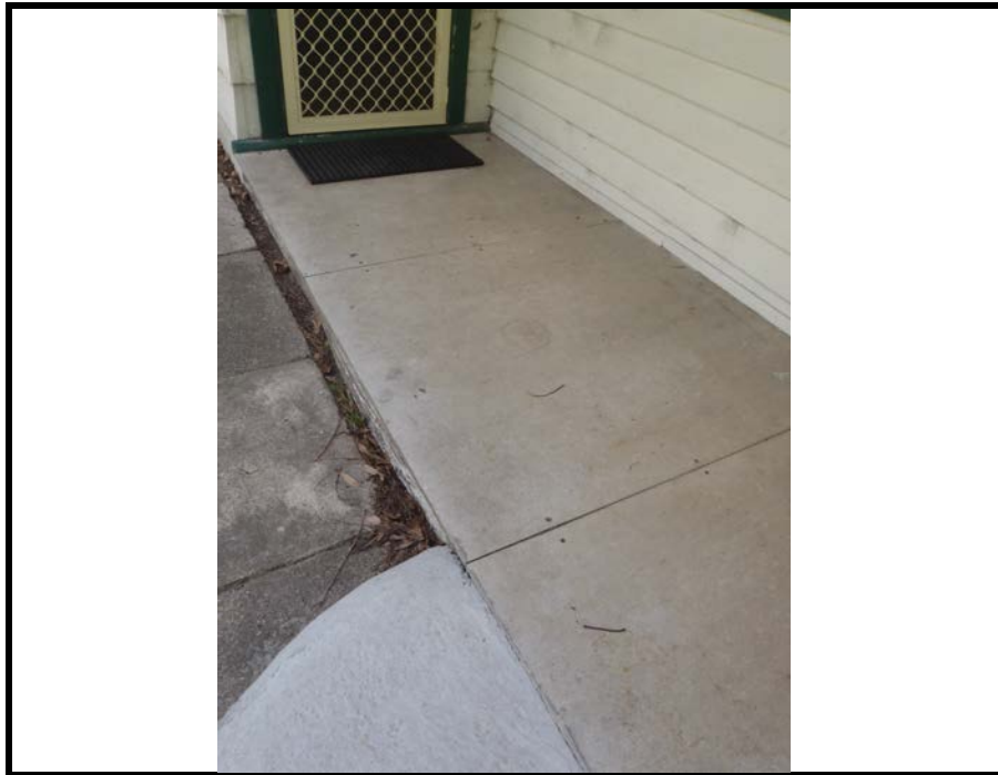
Photo 13: ACM sheeting used as flooring to the front awning of 2 Dawes Avenue
