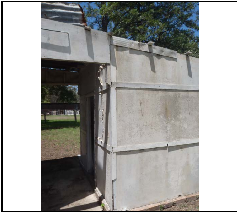
Photo 25: Exterior wall lining (including edge strips) to laundry/ shed at the rear of the house at 4 Dawes Avenue.
