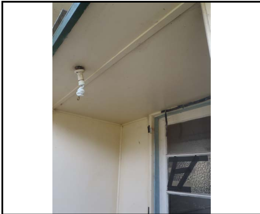
Photo 3: Example of ACM sheeting eaves and exterior walls to 1 Dawes Avenue
