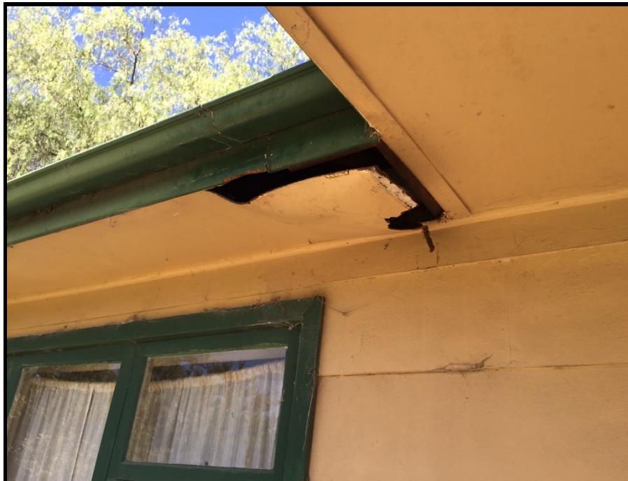
Photo 33: An example of the ACM sheeting boards used on the exterior of 8 Dawes Avenue.
