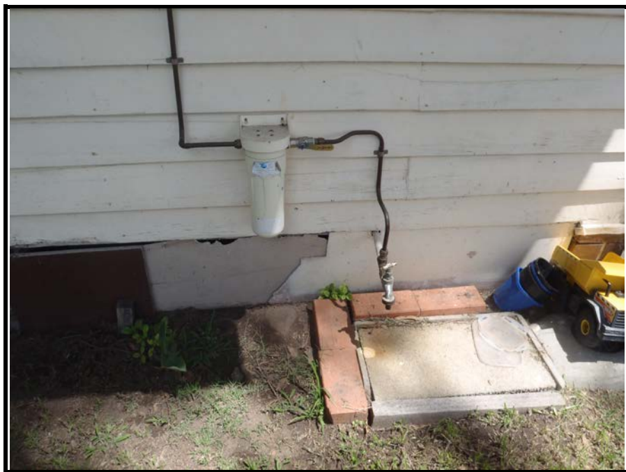
Photo 16: ACM sheeting used as infill panels below house at 2 Dawes Avenue (note: only this small section behind the tap)
