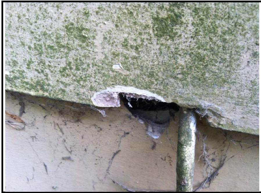
Photo 33: An example of the ACM sheeting boards used on the exterior of 8 Dawes Avenue.
