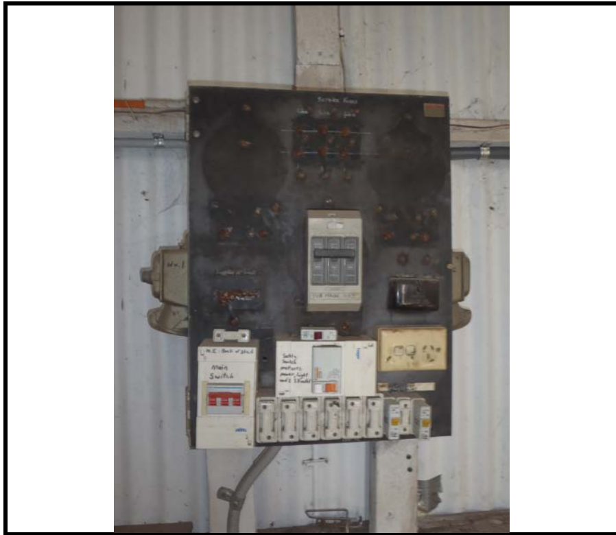
Photo 9: ACM backing board to power board in small shed at 1 Dawes Avenue
