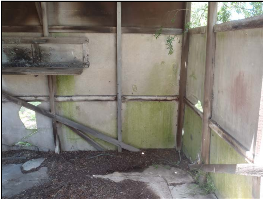
Photo 23: ACM corrugated sheeting used on garage at 4 Dawes Avenue
