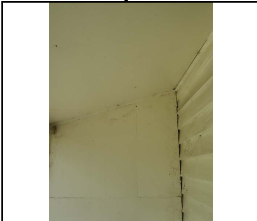
Photo 11: The metallic sheeting that is potentially lining SMF insulation to the roof of the large shed at 1 Dawes Avenue.
