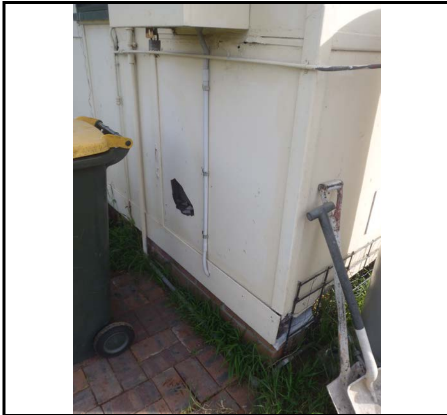
Photo 1: Example of ACM sheeting (and damage) to exterior walls of 1 Dawes Avenue
