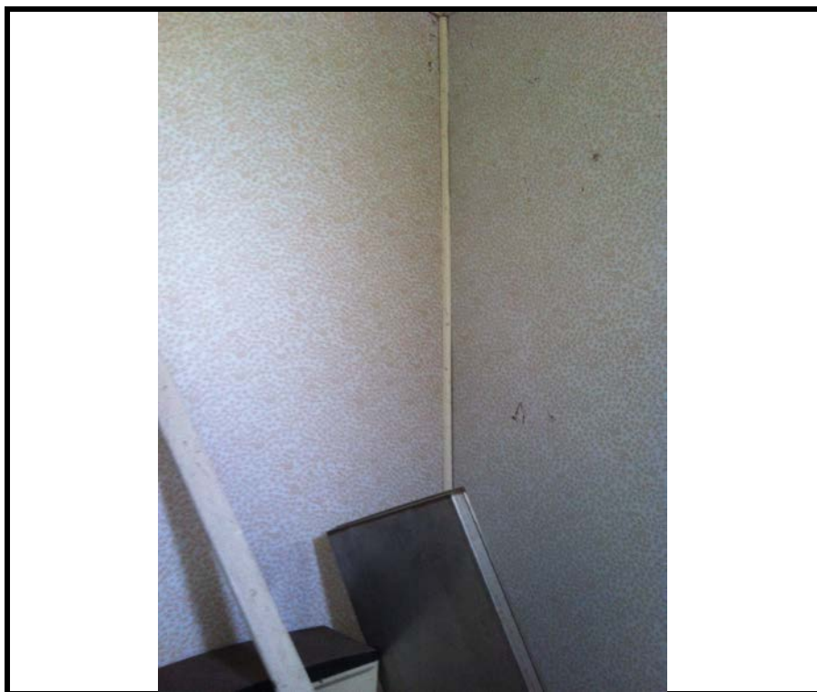
Photo 35: Section of ACM wall lining (lower section) to bathroom.
