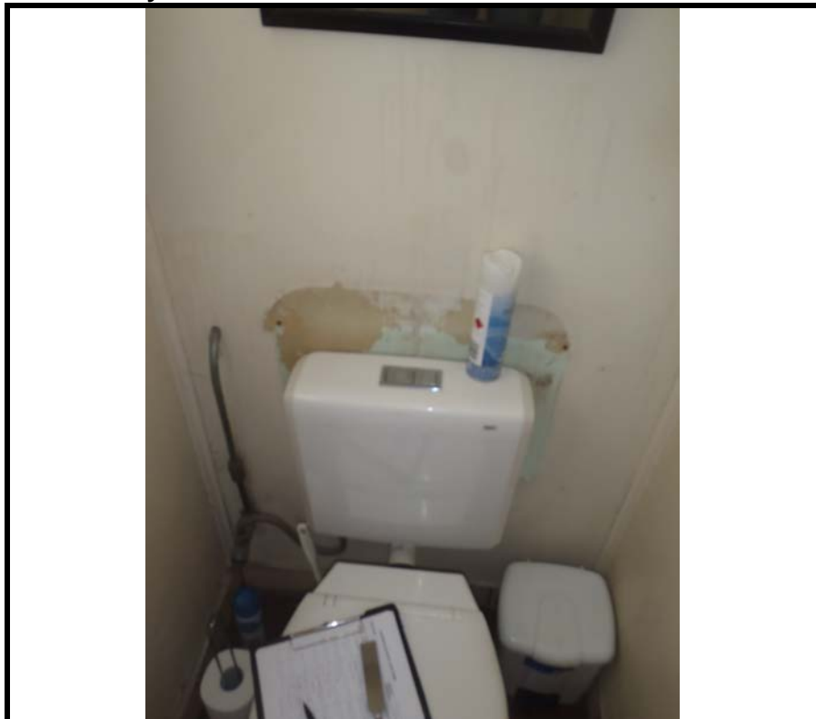
Photo 7: Section of the ACM sheeting walls to bathroom at 1 Dawes Avenue. Note mostly in good condition, some paint worn immediately above bath.
